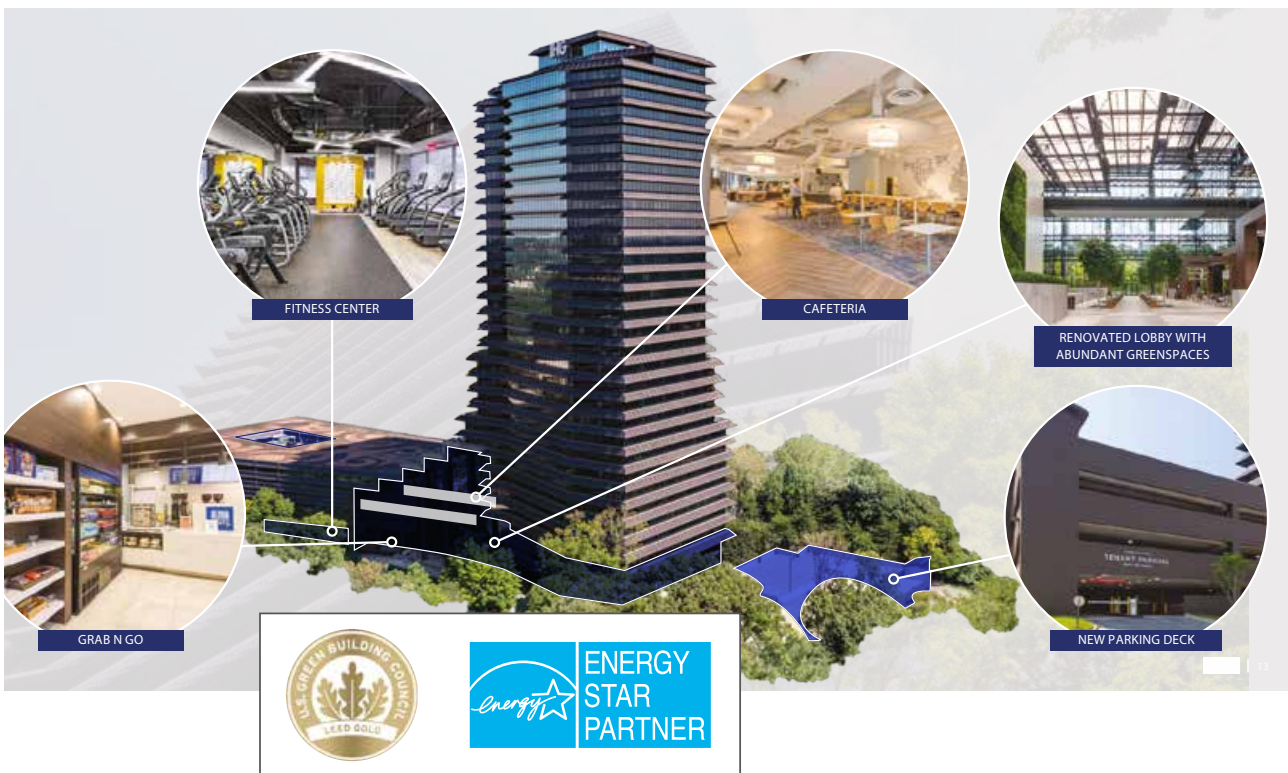
LEED Certification & Energy Star ratings
